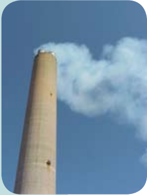
Coleson Cove Generating Station
