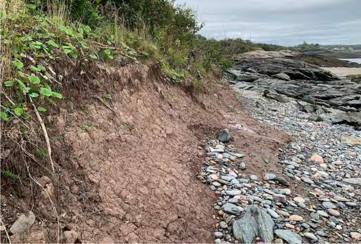
Figure 27. Massive clay bed eroding at waypoint 171, facing east.
