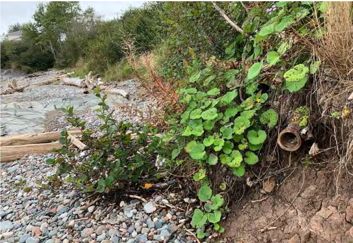
Figure 28. Clay bed with pipe on surface slump. Facing west at waypoint 171.
