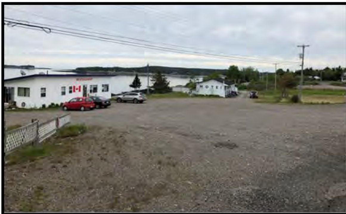
Photo No. 1: Project Site (all Buildings to be Removed or Demolished)
