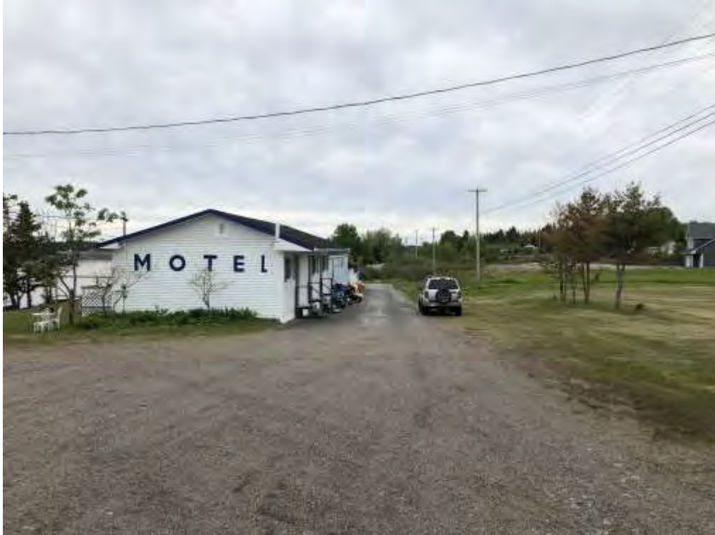
Photo No. 6: Motel
