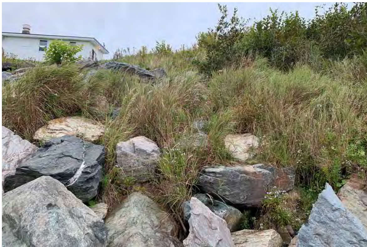
Figure 21. Facing upslope from waypoint 168, armour stone installed by owner.
