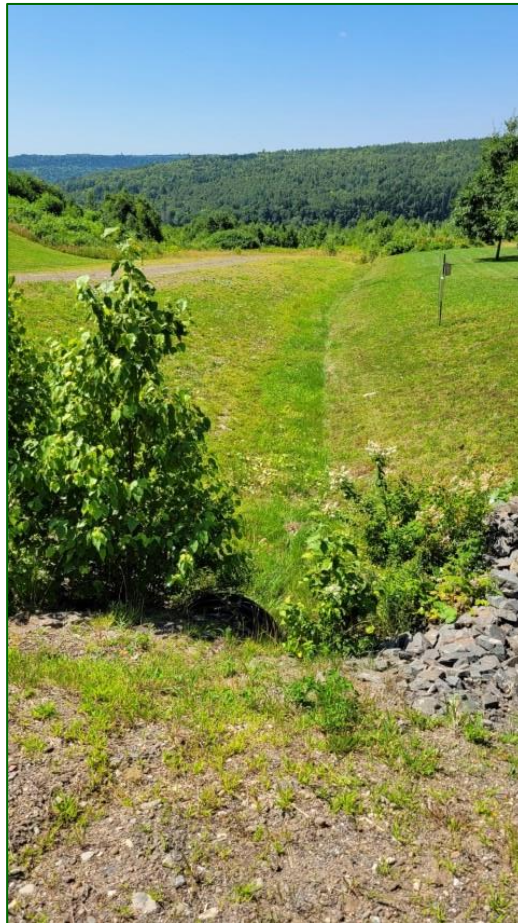
FIGURE 7. DRAINAGE DITCH TO THE WEST OF INSPIRATION LANE THROUGH WHICH DRAINAGE FROM WETLANDS 3, 4, 5, 6, AND 7 FLOWS TOWARDS THE NASHWAAK RIVER.
