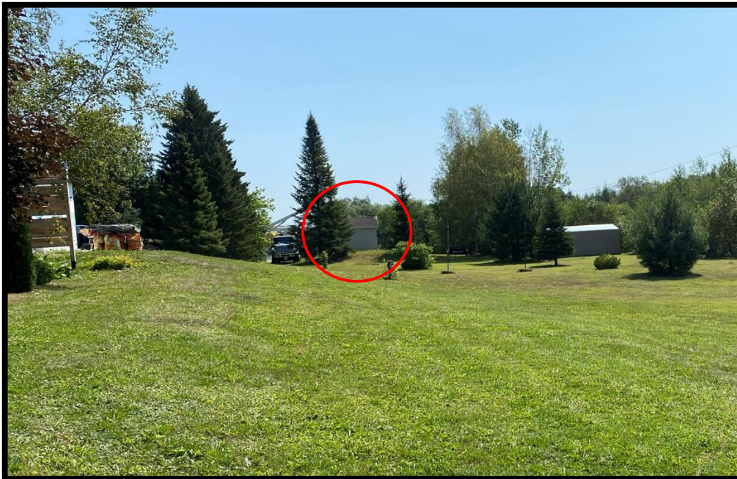
Photo No. 3: Rita Smith Street Well to be Decommissioned (in red circle)
