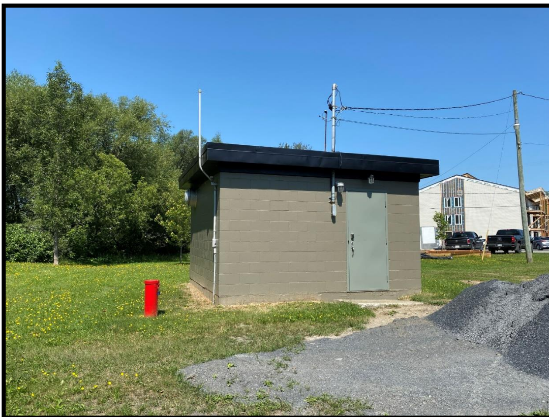
Photo No. 1: Jos-Soucy Pumphouse and Observation Well, Site of RW1
