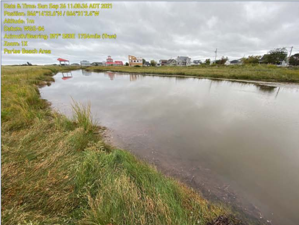
Photograph 34. Dredging Area B, facing east.
