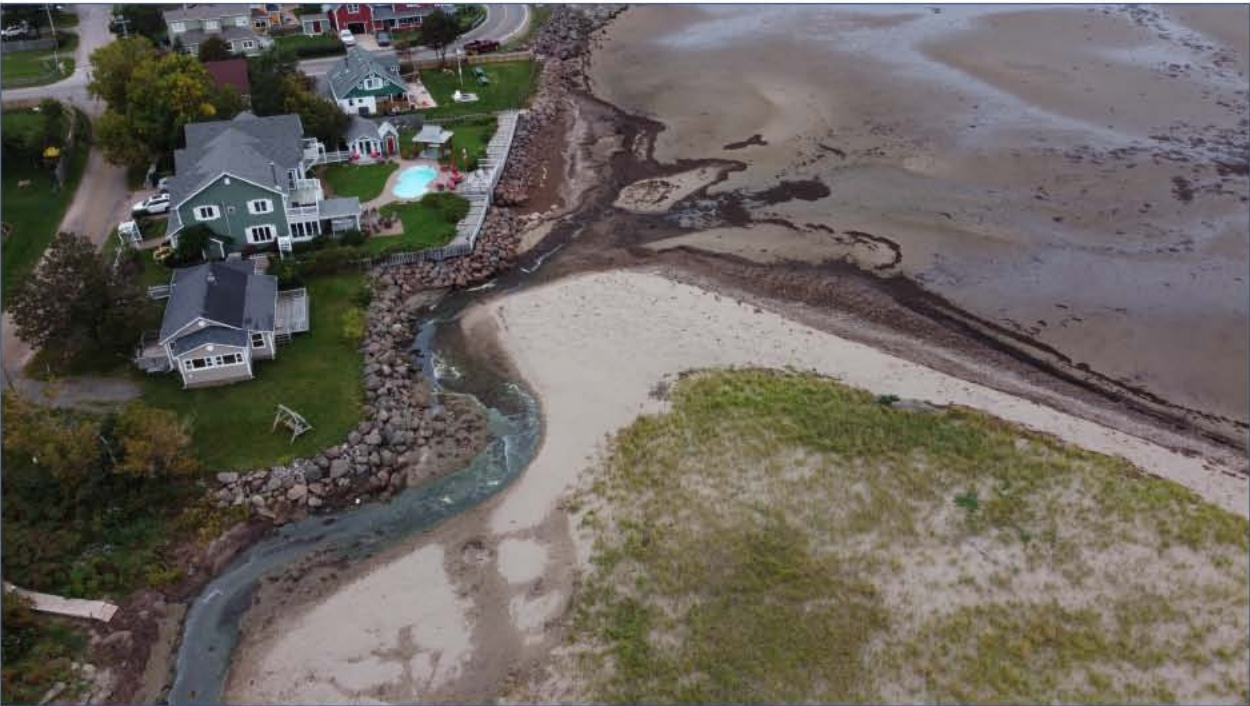
Photograph 51. Overview of Dredging Area A.
