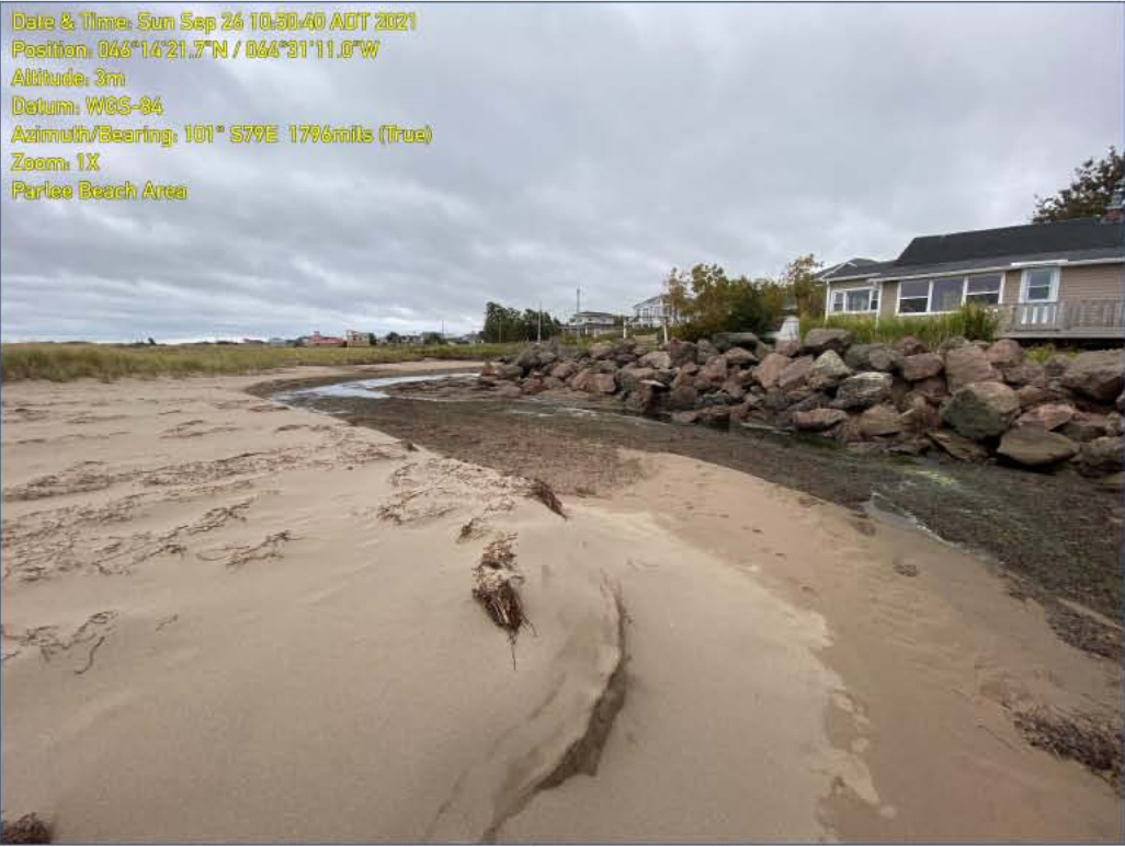
Photograph 29. Dredging Area A, facing east.
