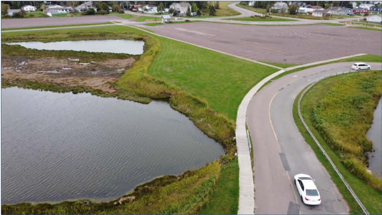
Photograph 57. Road and corrugated steel pipe culvert at filled causeway, at Dredging Area D.
