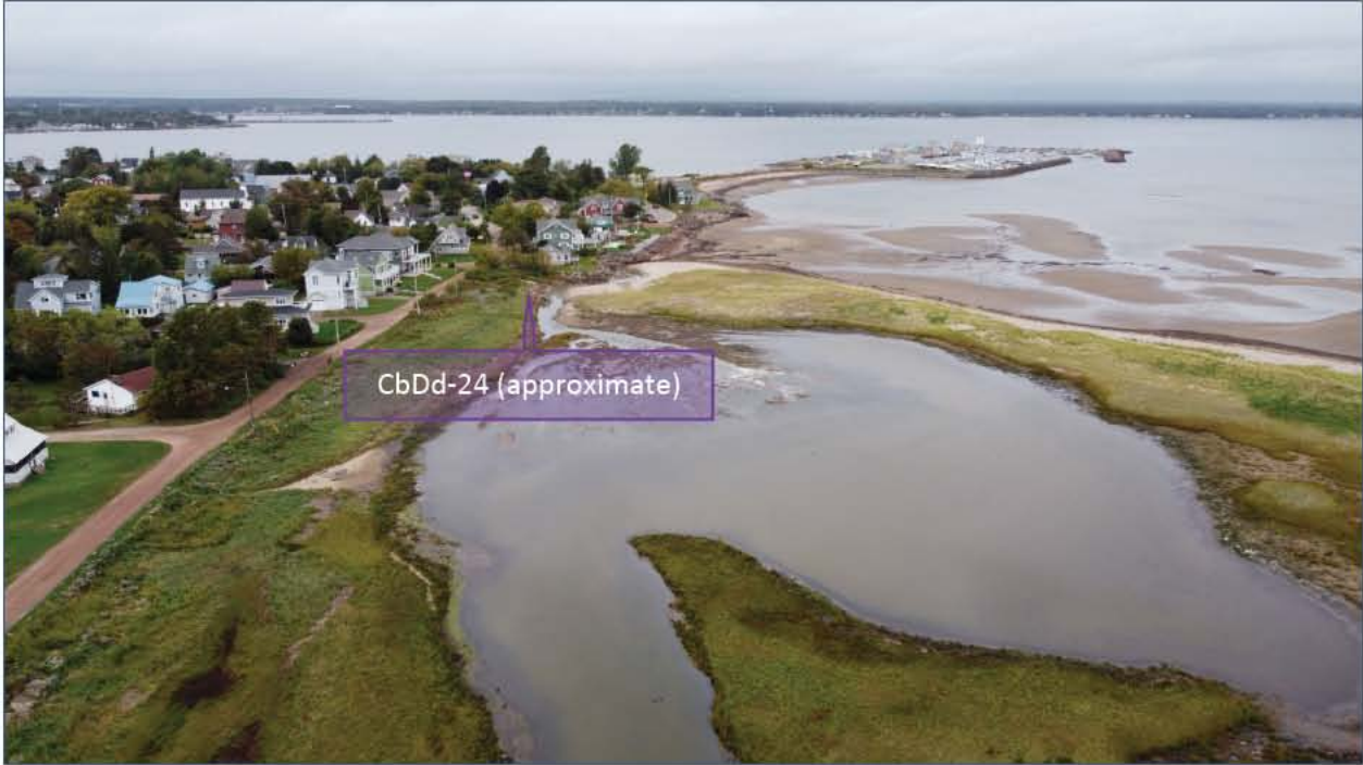
Photograph 48. Overview of Dredging Area A in background with Dredging Area B in foreground.
