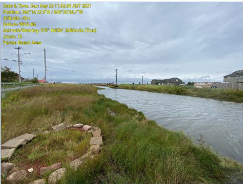
Photograph 39. Facing west towards Dredging Area C.
