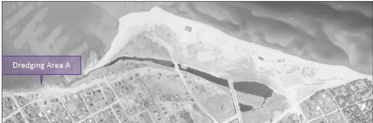
Photograph 14. Excerpt from 1971 aerial photograph Project Area.
