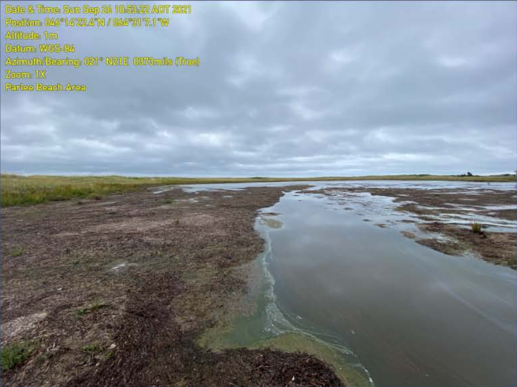
Photograph 32. Dredging Area A, facing north.
