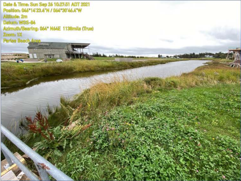
Photograph 24. Dredging Area C, facing east.
