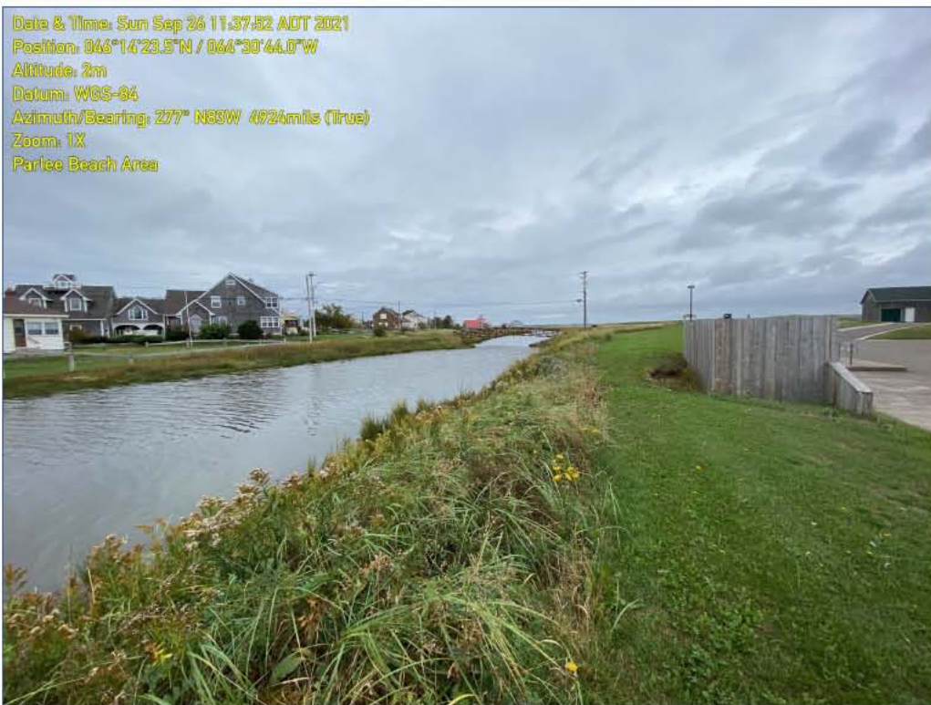
Photograph 35. Dredging Area C, facing west.
