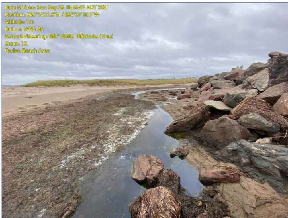
Photograph 19. Western end of Project Area, dredging Area A, facing east.
