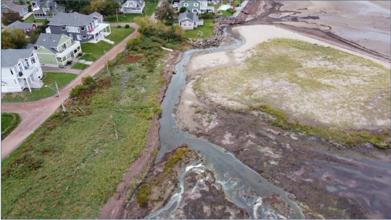
Photograph 50. Overview of Dredging Area A.
