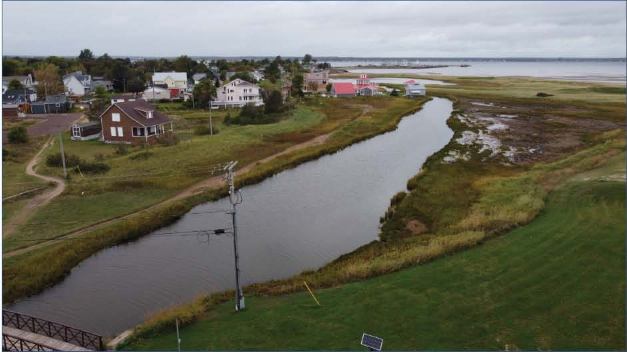
Photograph 53. Part of Dredging Area C, foreground, facing towards Dredging Areas A and B.
