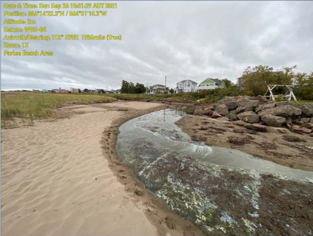
Photograph 30. Dredging Area A, facing east.
