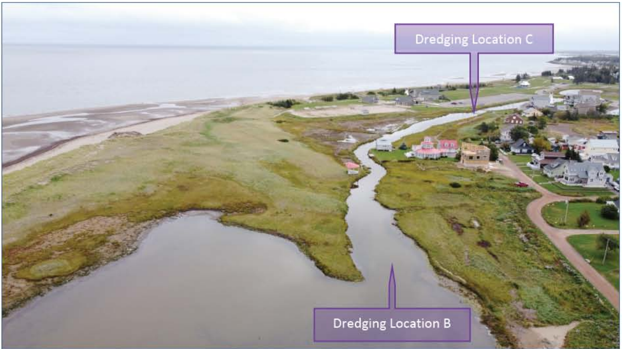
Photograph 45. Dredging Area B and Dredging Area C.
