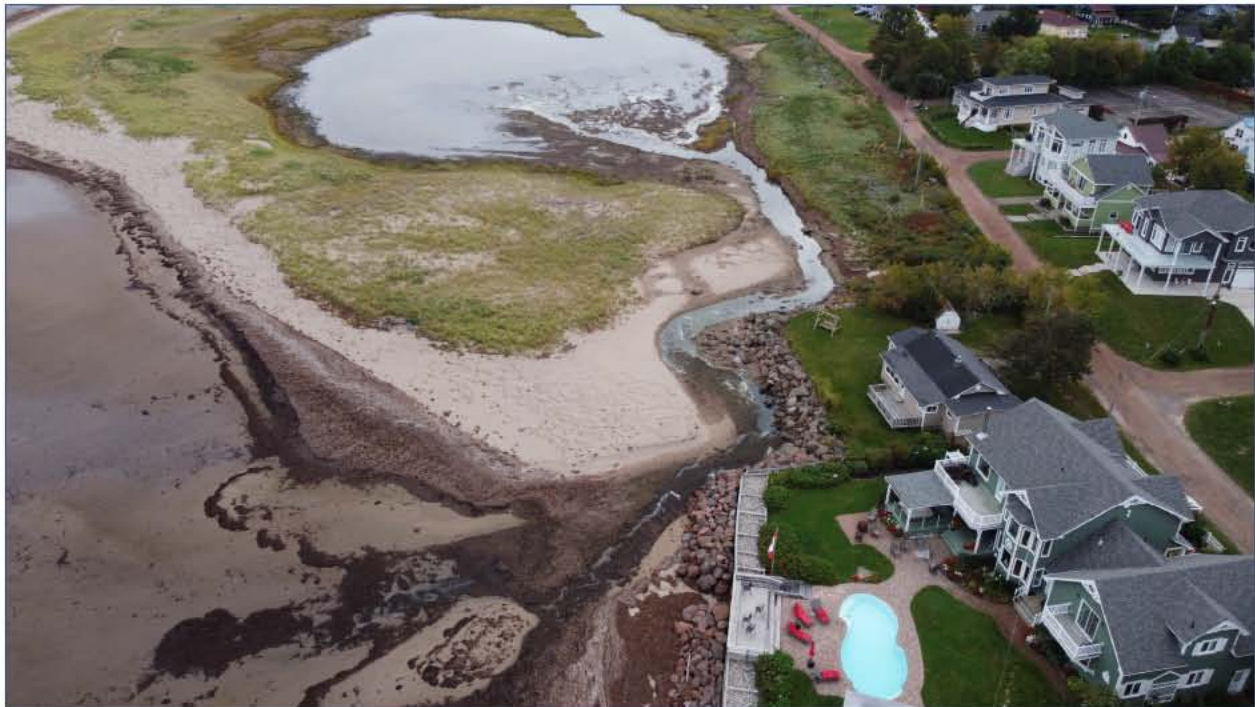
Photograph 43. Overview of Dredging Area A with Dredging Area B at top.
