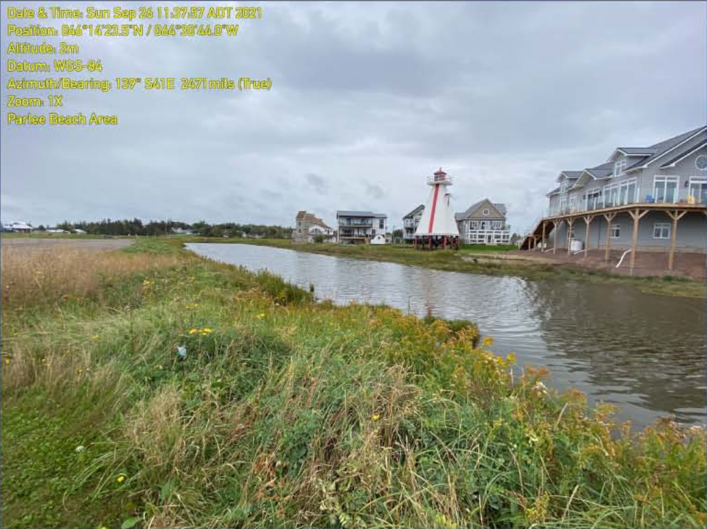
Photograph 36. Dredging Area C, facing west.
