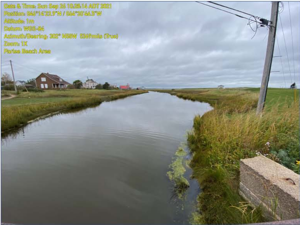
Photograph 25. Dredging Area C, facing west.
