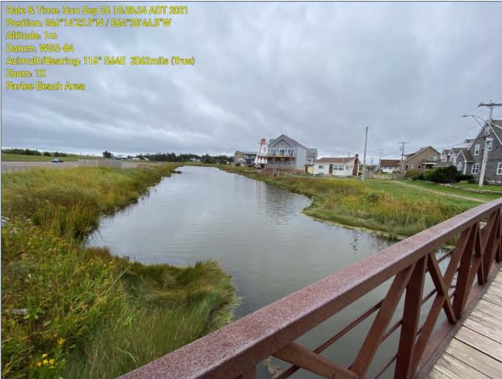
Photograph 26. Dredging Area C, facing east.
