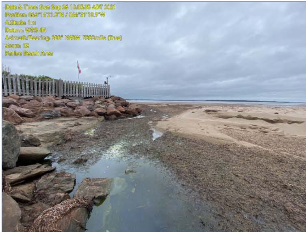
Photograph 18. Western end of Project Area, dredging Area A, facing west.
