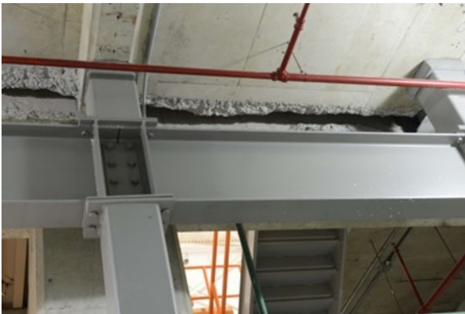
Figure 2.2 Effects of AAR at the Mactaquac Generating Station
