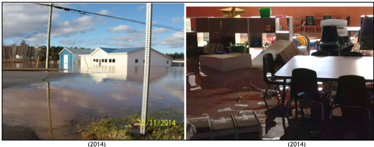
Figure 1: Examples of Past Flooding - Fox Creek Area, Dieppe, N.B. 1 2
