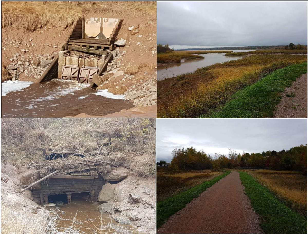
Figure 2: Photos of Existing Aboiteau Structure and PSW
