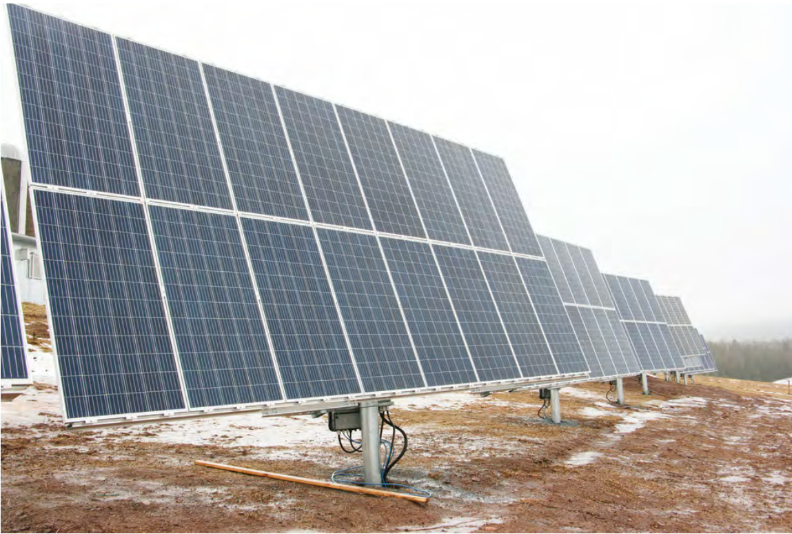
Figure 9. Photograph showing some of the ground-mounted tiltable solar panels at the Auenland Dairy Farm in Mount Pisgah, New Brunswick.
