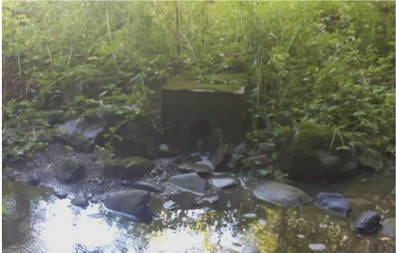
Photo No. 2: Lagoon Outfall Pipe
