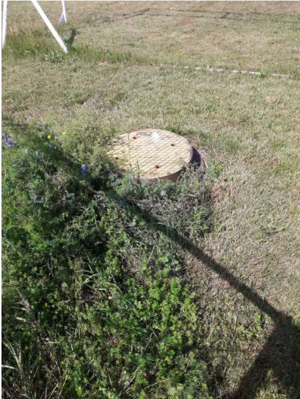
Photo No. 3: Manhole at Sports Field
