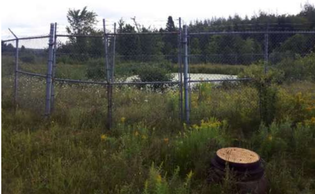
Photo No. 8: Lagoon Gate, Manhole
