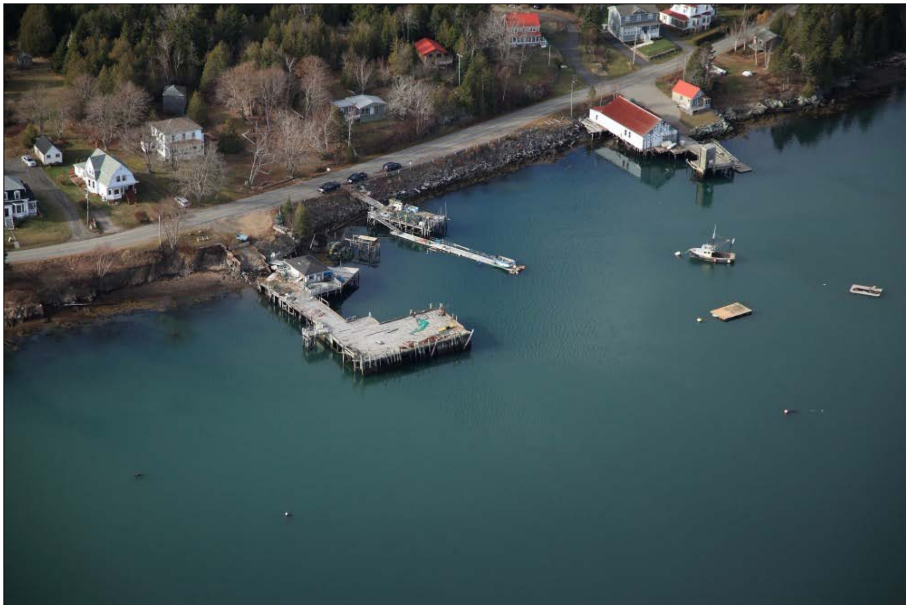
Figure 7: Aerial Photograph, Richardson Wharf DFO-SCH, Deer Island, New Brunswick (18-Nov-2017)
