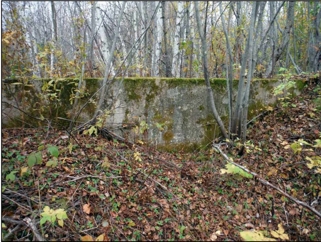
Figure 6: Portion of large concrete foundation at south end of development.
