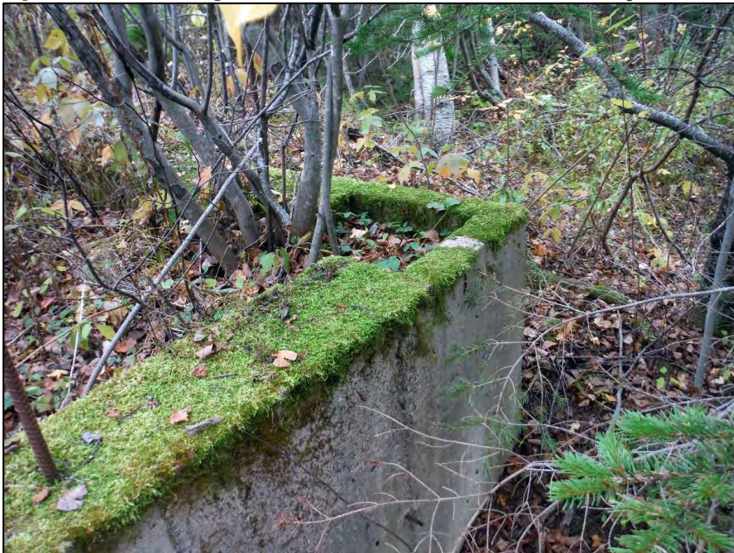
Figure 7: Portion of large concrete foundation at south end of development.
