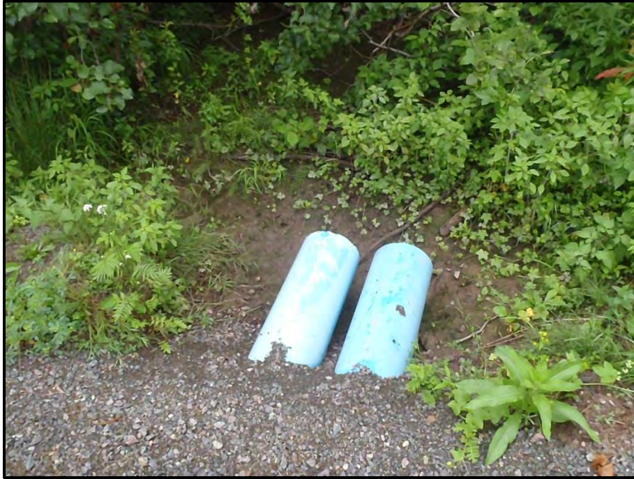
Photo 9 – Dry upstream side of culverts crossing trunk line.
