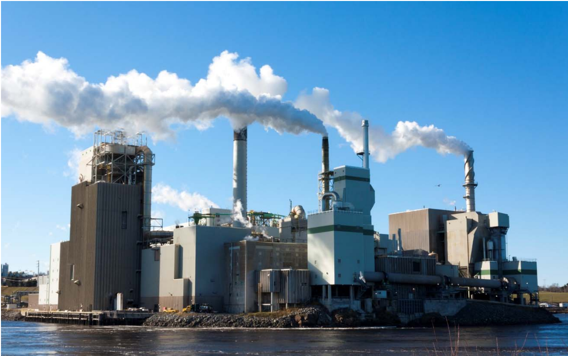
Figure 4. The Irving Pulp & Paper, Limited Reversing Falls Mill located near the mouth of the Saint John River in Saint John, New Brunswick.
