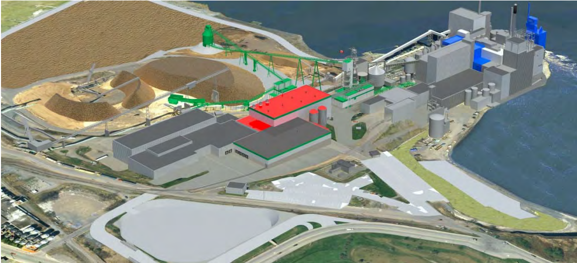
Figure 8. Three-dimensional model looking northwest showing three phases of the long-term multi-phase upgrade program at the Reversing Falls Mill in Saint John, New Brunswick. Phase 1, new lime kiln and pulp washing equipment upgrade, is shown in blue, Phase 2, new chip handling processes and continuous cooking digester plant renewal, is shown in green, and Phase 3, pulp dryer modernization, is shown in red.
