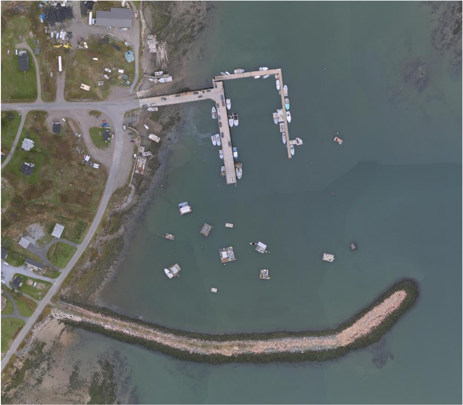
Figure 3: Oblique aerial photo of Back Bay Small Craft Harbour, Charlotte County, New Brunswick.
