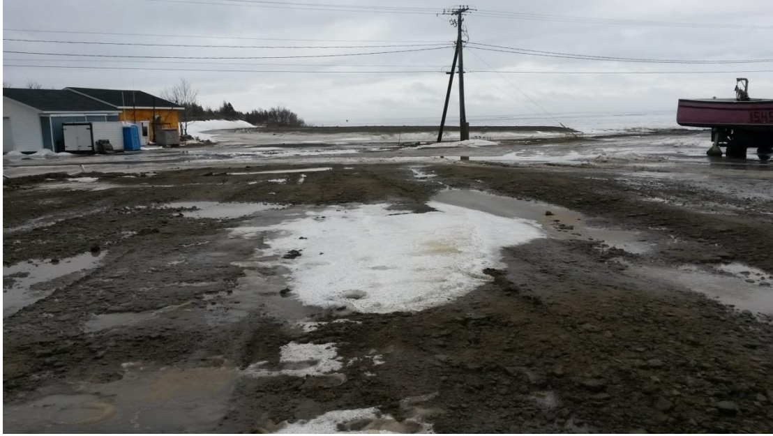
Photo no. 3: Construction footprint east of existing structure.
