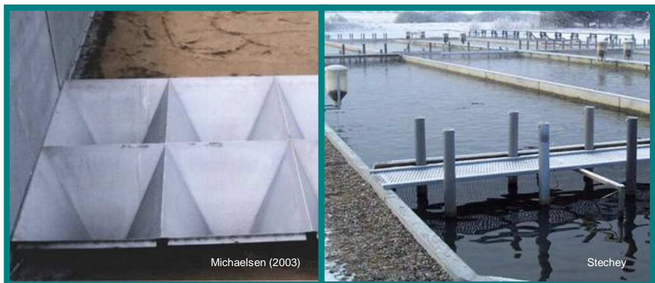
Figure 15: (L.) Sludge cones being installed in a raceway. (R.) Standpipes extending from sludge cones in a Danish raceway
