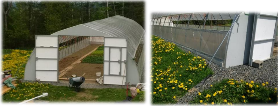
French drains: gravel and perforated drainage pipe
