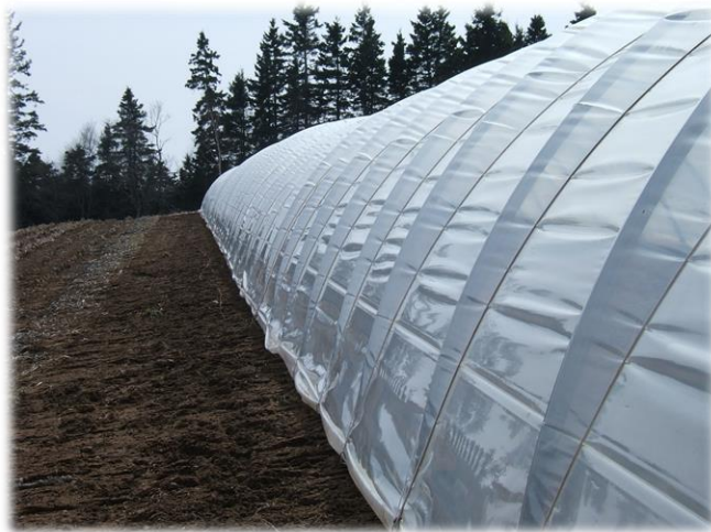
View of lacing rope
