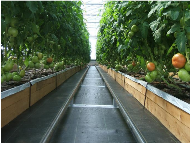
Pipe network used to circulate hot water and to carry the utility carts
