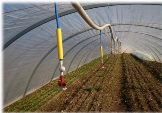
C. tunnel with over-head sprinklers great to encourage germination and for the production of greens
