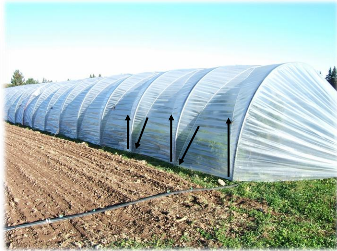
View of lacing rope
