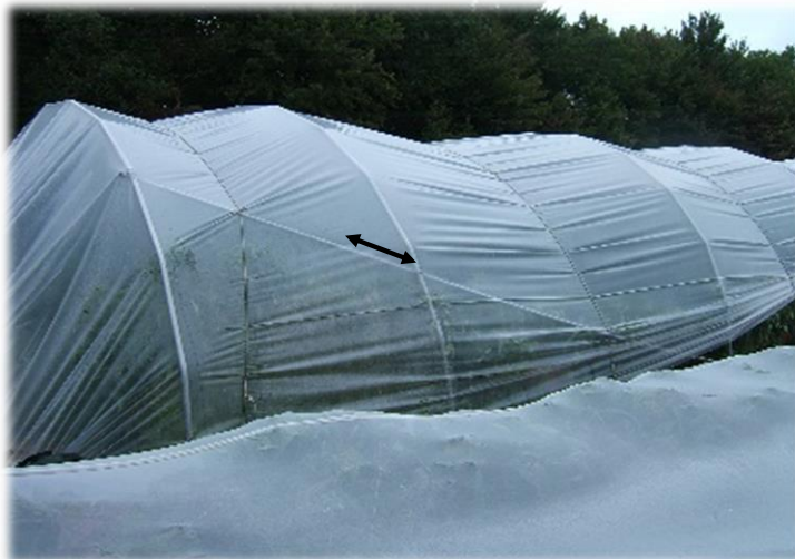
C. tunnel with 4 diagonal stiffeners to add stability at the ends of the structure
