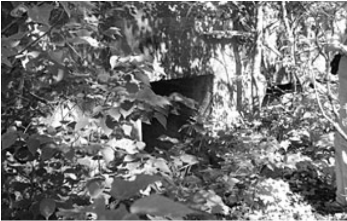
Figure 3.2 - View of the exterior of Bunker OP-1 (CiDg32).
