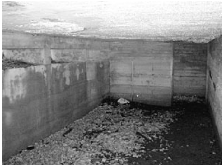
Figure 3.4 - View of interior of Bunker OP-8 (CiDg33).
