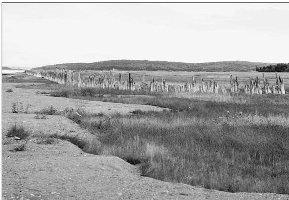
Figure 7: Upright log curtain running parallel to the small earthen dykes in the marsh just north of the Rocks Park entrance booth (1994).
