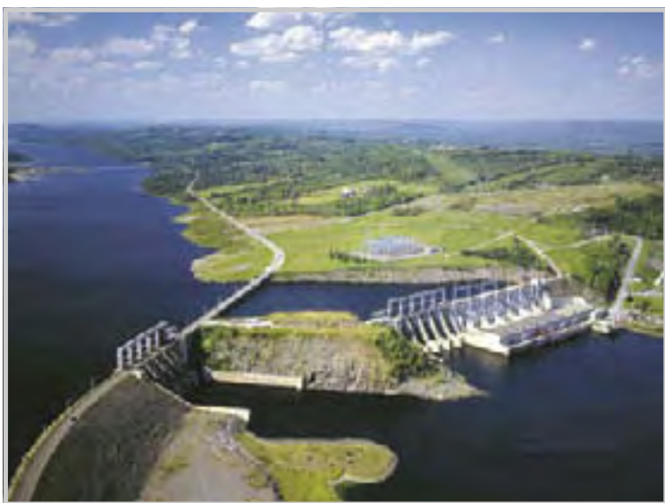
A view of the Mactaquac hydroelectric dam with Keswick Ridge rising behind it. The ridge is underlain by slightly calcareous sedimentary rocks. Photograph © Ron Garnett–AirScapes.ca.
