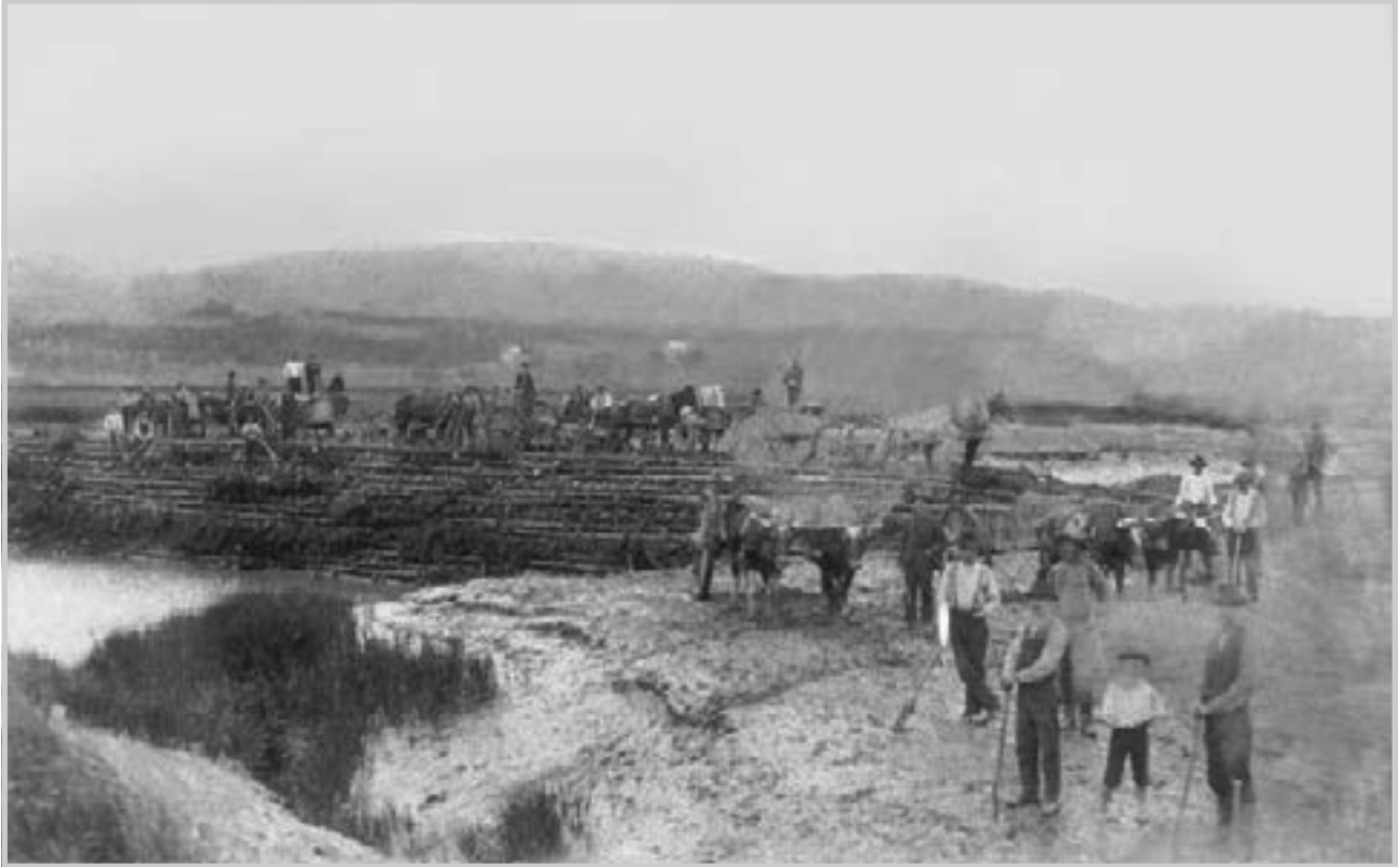
Acadian dike building, ca 1880. Photograph courtesy of Université de Moncton library archives.
