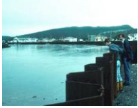
Seawall at Placentia, Newfoundland and Labrador
