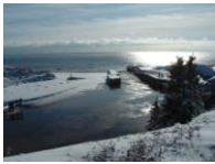
Infrastructure Damage, Basin Head Provincial Park, PEI
