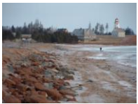
Storm Surge Damage, Panmure Island Causeway, PEI
