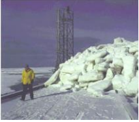
Ice Damage to Wharf, Aboiteau Wharf, NB
