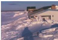
Ice Damage, Maximeville, PEI
