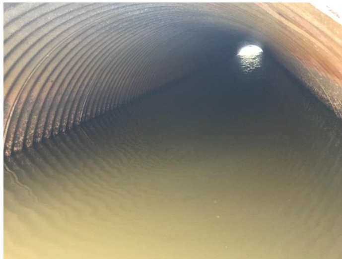
Figure 4-1: Inside Photo of Central Culvert
