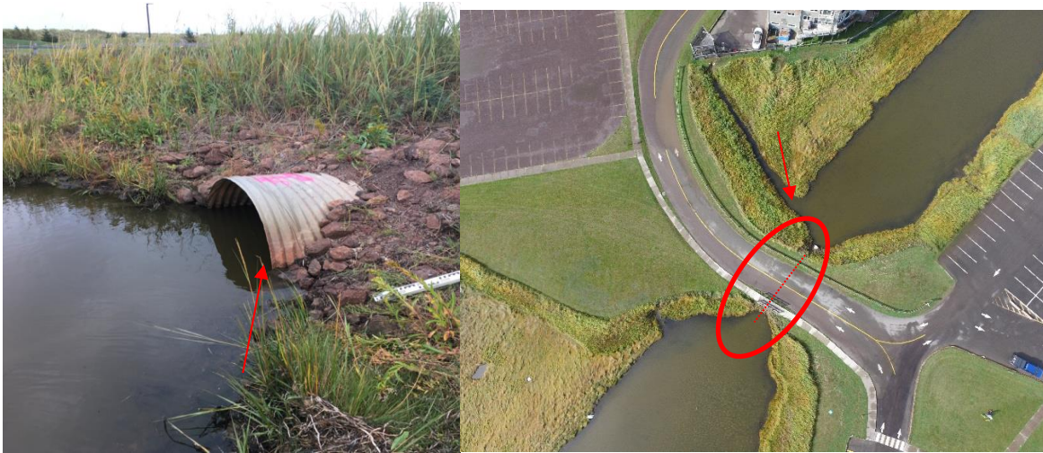
Figure 2-3: Culvert no. 1 (1200mm Diameter Corrugated-Steel Pipe (CSP))
