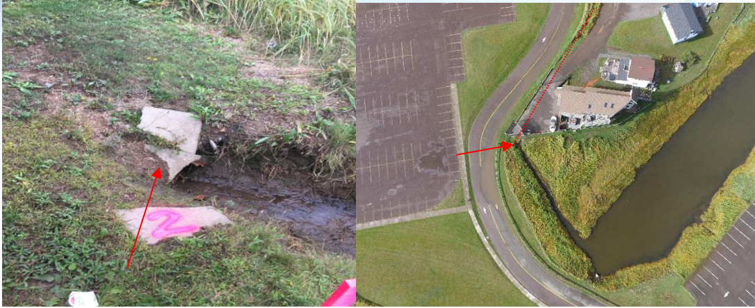
Figure 2-4: Storm Outlet No. 2 (350mm Diameter CSP)
