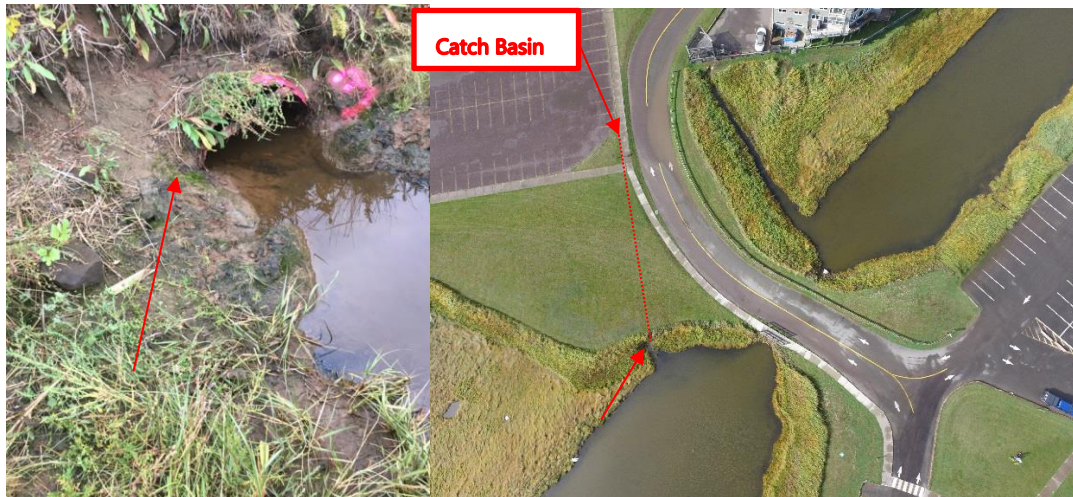
Figure 2-5: Storm Outlet No. 3 (750mm Diameter CSP)
